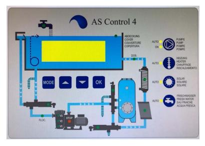
(Filter) Pump AUTO/ON/AUS Trigger a Backwash cycle
